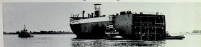
MOVING BY WINCH AND GRAPPLE LAST SUMMER —As soon as the sea was still, the body had been placed, elongated steel trussing upriver for #2 dry dock. . . .
