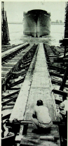
FRONT OF ANOTHER colossal floating iron chest as THE EXPORT COMPANY , completely unsharpened, starts to swing up-line toward waiting tugs.
