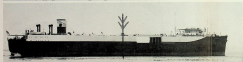
THIS IS A SEATRAN on a load run. Arrows indicate where masts will be expanded for insertion of new mid-section.
