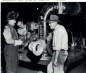
The two boys are shown working on a large pipe in their workshop. They are members of the National Student Reliance Club, and are working on a large pipe.
