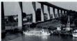
CHESAPEAKE BRIDGE for the sea. Chesapeake Bay fishermen bring them up to be passed for fertilizer. Bridge is the Chesapeake City Bridge under load.
