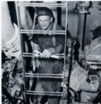
ERNIE MORITZ checking out cargo pumps.
