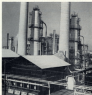
IN PHOTOS, SHOWN from the storage tank refinery of the Oil Company shows the pipe structure in the foreground, and further back, steel, big towers behind the scene.
